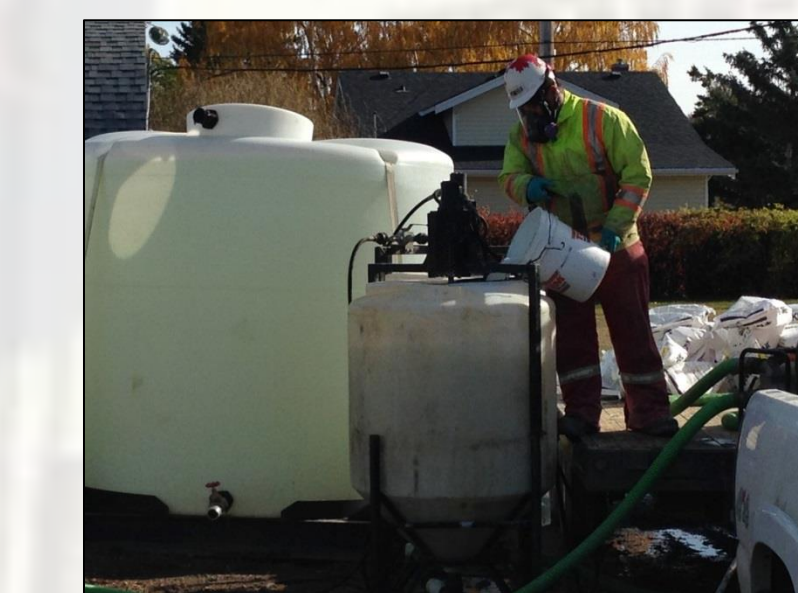
Mixing of NaOH activator with persulfate
