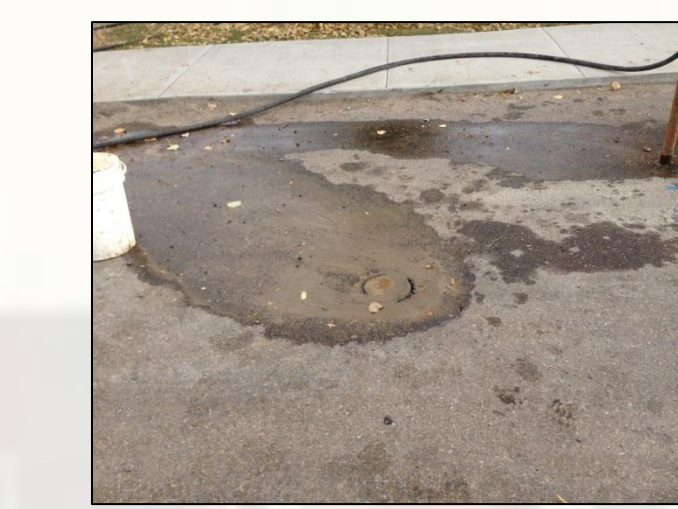
Daylighting of persulfate within adjacent monitoring well
