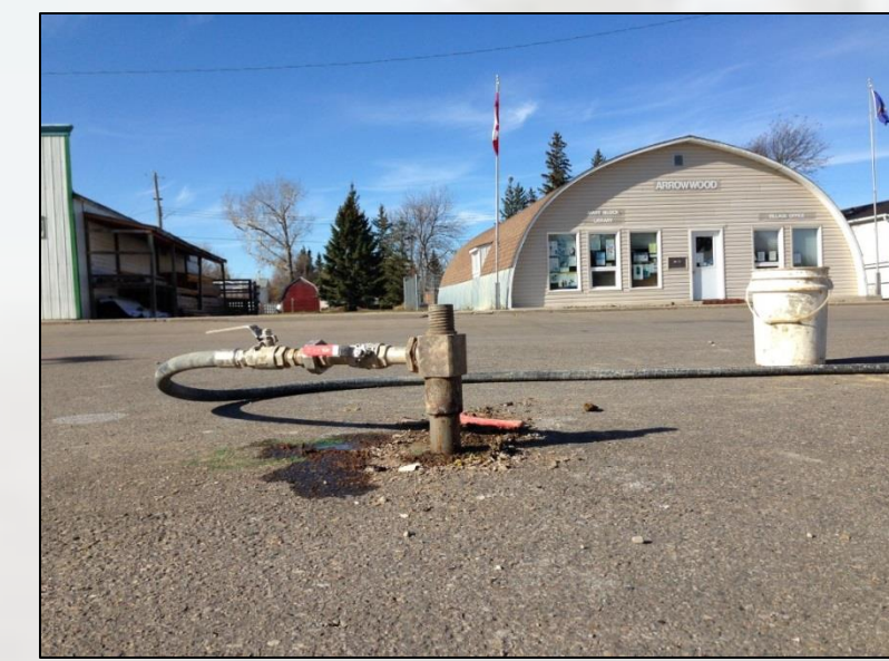
Injection rod and transfer hosing installed within investigation area
